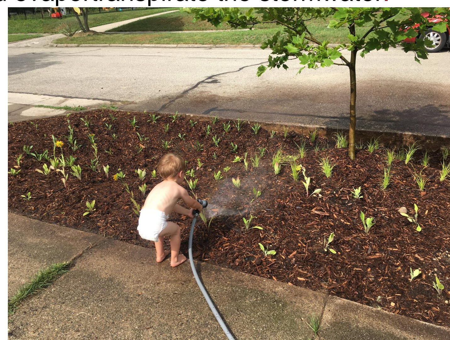
Fig. 1: A curb-cut rain garden installed by Plaster Creek Stewards being watered by a dedicated volunteer.
