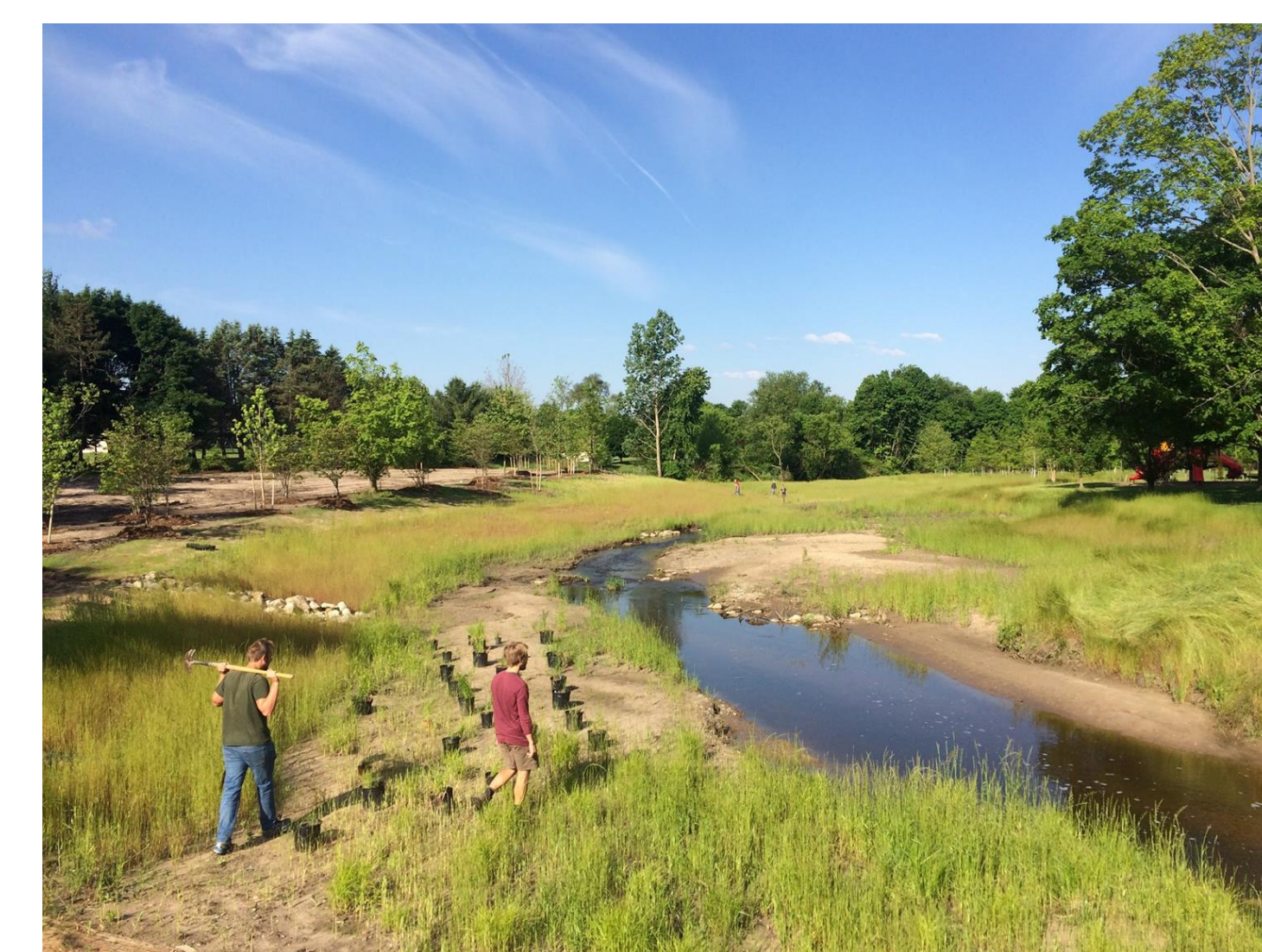
Fig. 4: Shadyside Restoration Project located at the headwaters of the Plaster Creek watershed.
