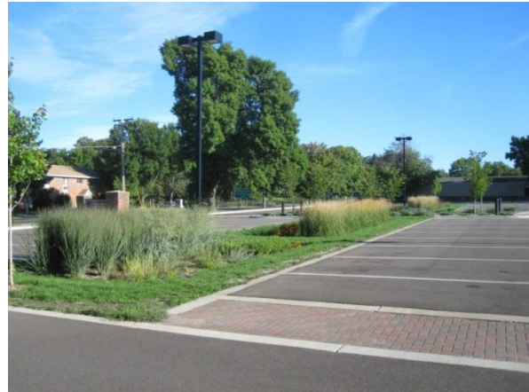
Figure 5-2. Bioretention example in parking lot.
