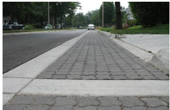
Figure 5-3. Porous pavement example.
