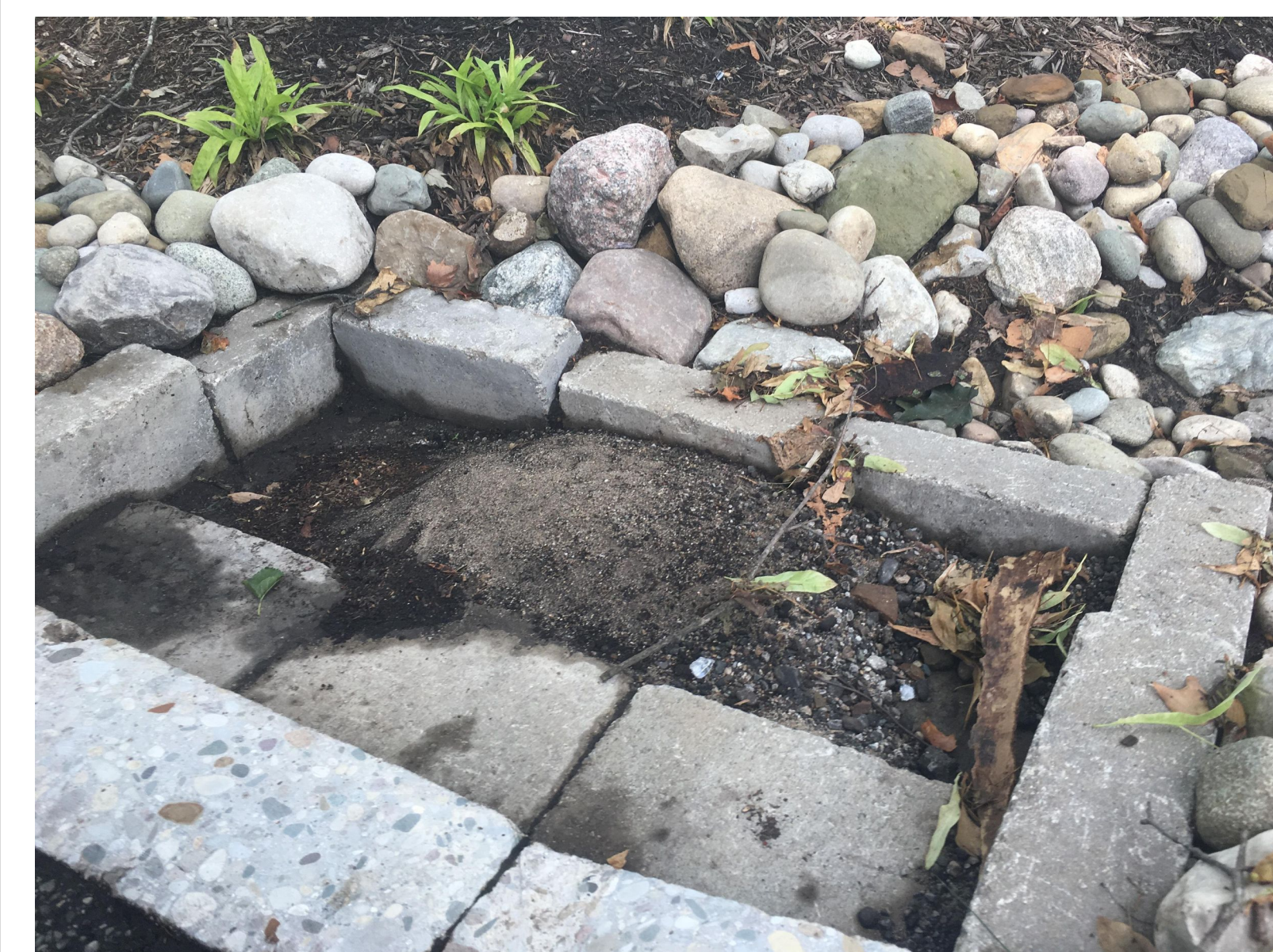
Fig. 3: A sediment trap in a rain garden filled with sediment. The sediment was deposited by stormwater moving through the trap
