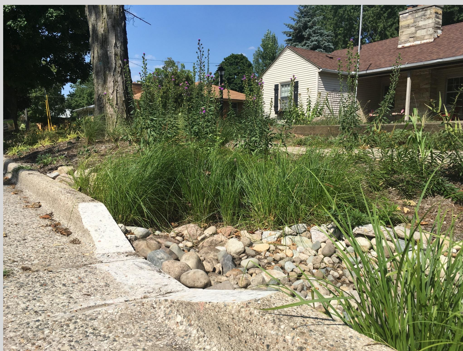
Figure 1: The curb cut of a two year old rain garden on Linden Ave. in Alger Heights, MI
