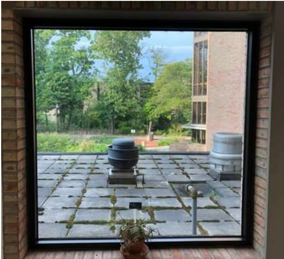
Figure F1. 1: Base Case Devries Hall APW5050 double pane window. EE case includes same window except with three panes and SmartSun Heatlock enhancement (model number is the same).
